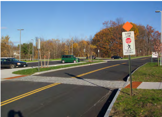
Example of pedestrian crossing with traffic calming on a campus road
