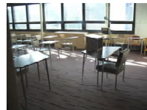
Priority 4 Example Replace worn interior finishes
