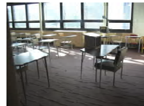
Priority 4 Example Replace worn interior finishes
